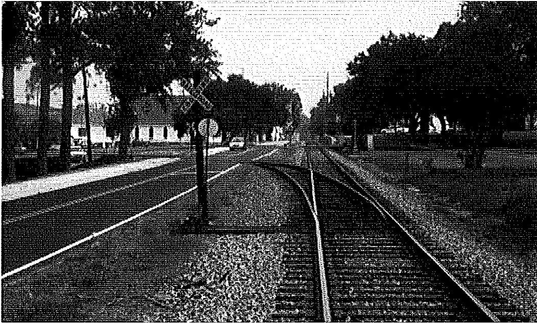
Figure 4. Looking north at the switch and turnout from the NS R main line onto the Avondale Mills industry track at Graniteville. The switch banner, or target, shows white, indicating that the switch is in the "normal" position, that is, aligned for movement along the main line track. (The banner shows red when the switch is set for the industry track.) North of the turnout and to the right of the main line is the wayside light indicating the position of the switch for the Vaucluse Siding.
